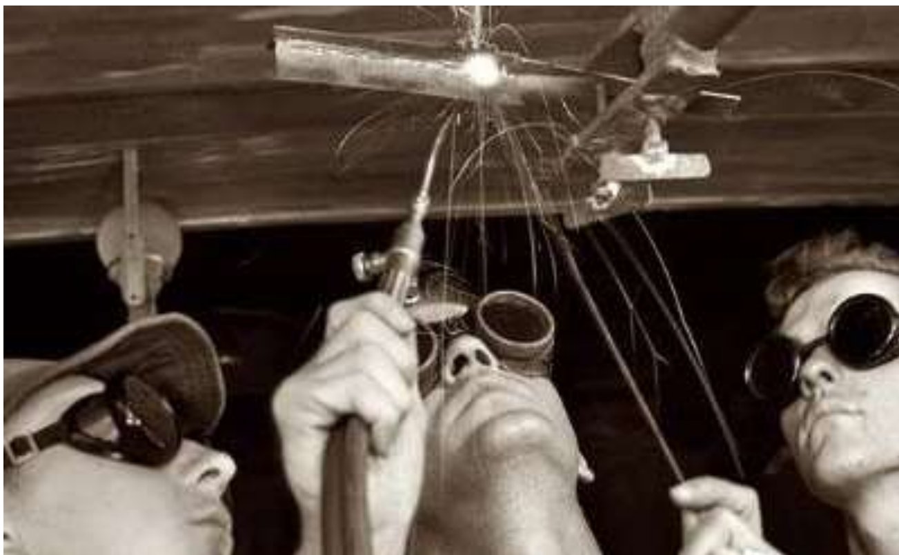
Building installation piping
